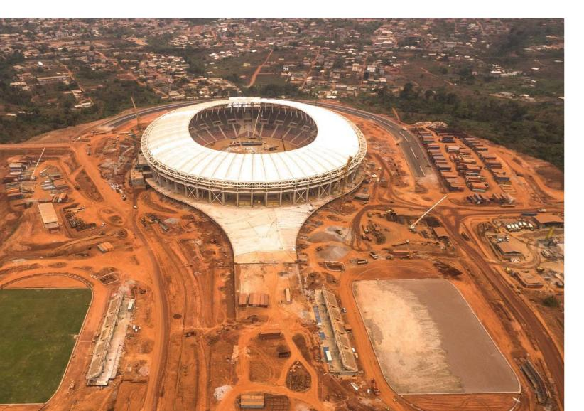
cables rather than by the inertia of each single element. This stadium typology permits a light and flexible structure, reducing installation time and crane capacity requirements. The rest of the structure is composed by prefabricated
