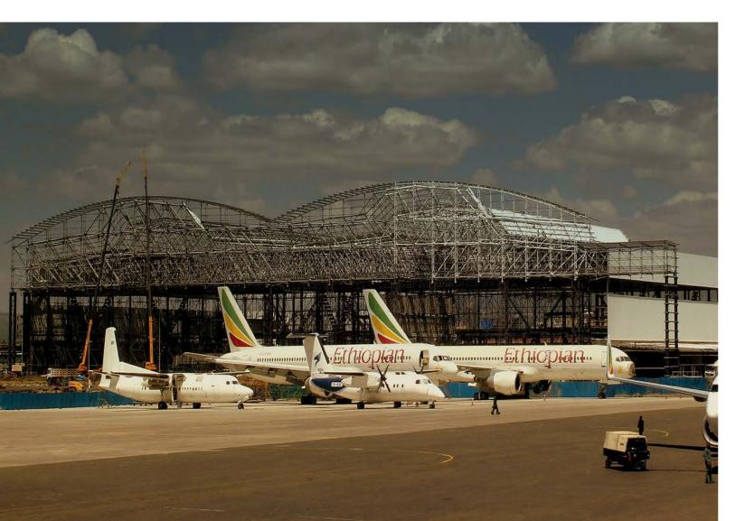
supporting structure of these buildings, with a total weight of 1.680 tons.
